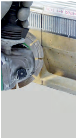
cutting the channel body to size
