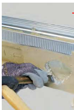
knocking out the recess
