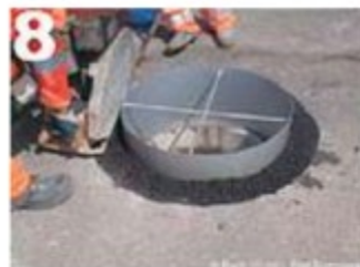
8 compacting asphalt
