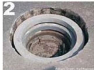
2 adjustment of adapterring and sandwichring
