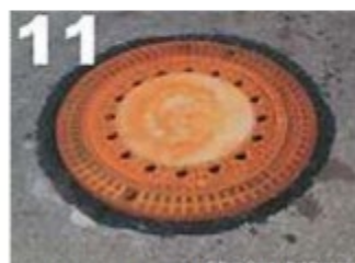
11 seal the manhole frame with the cover
