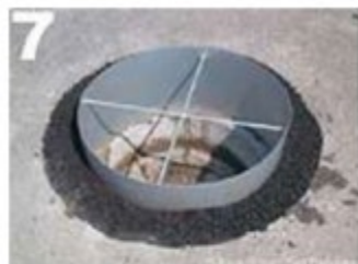
7 fill up workspace with asphalt
