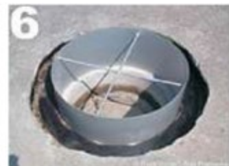
6 installation of bitumen shutter
