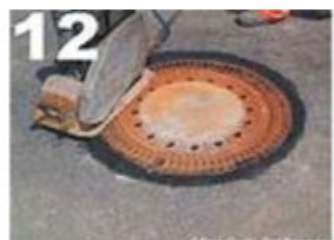
12 compacting to finished road level
