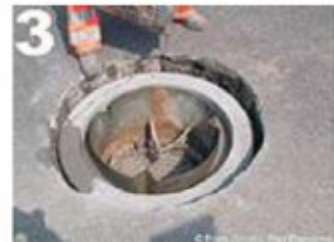
3 insert shutter and diffuse Ebralit®
